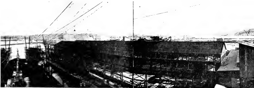
It will be noted that the main shop buildings parallel the building-ways on either side, the material movement from fabricating shops to ship hulls being direct.
